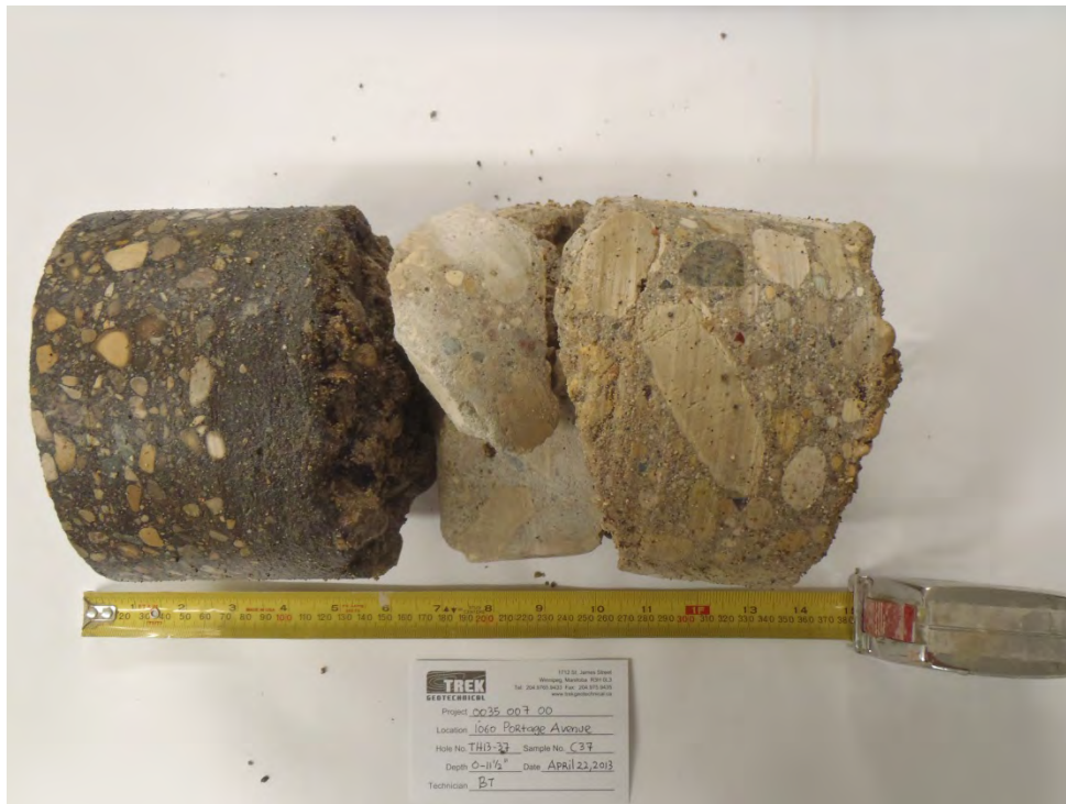
Photo 44: Asphalt and Concrete Core Sample from Test Hole TH13-37B
