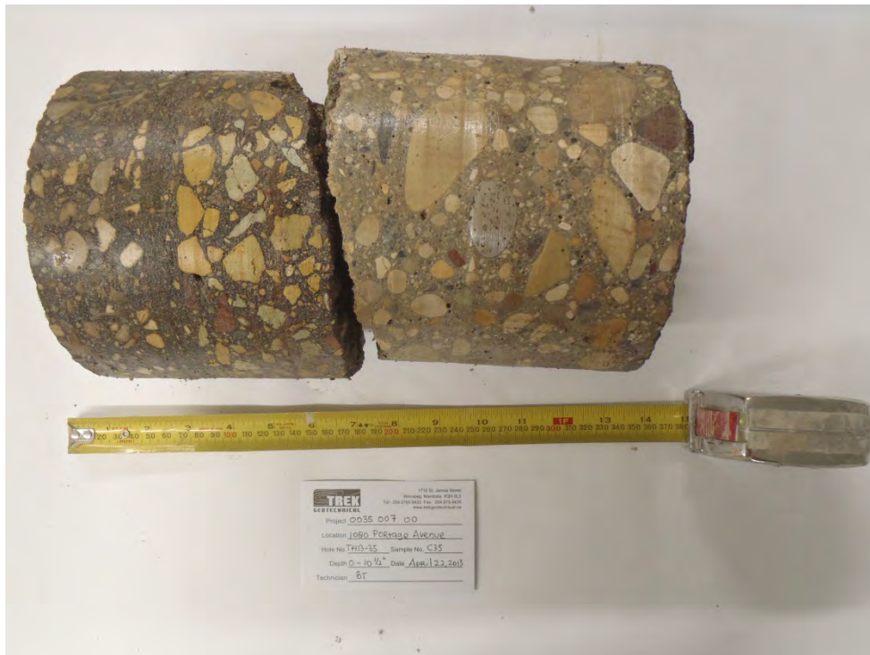
Photo 42: Asphalt Core Sample from Test Hole TH13-35B
